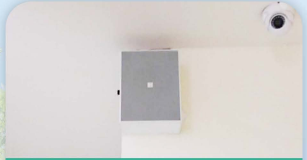
Replacement of Hospital Paging System Speakers January 1, 2025
