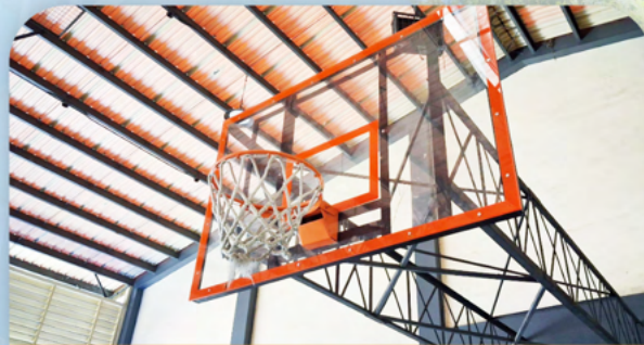
Installation of Basketball Fiberglass Board April 1, 2025
