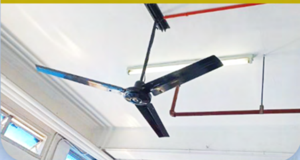
Installation of 18 Units Ceiling Fans at Doctors Clinics Waiting Area March 1, 2025
