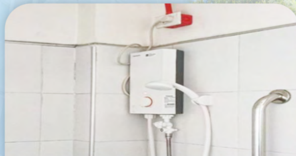
Installation of Shower Water Heater at Service Wards March 1, 2025
