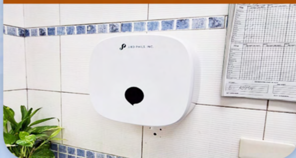
Installation of Jumbo Roll Tissue Dispensers May 1, 2025
