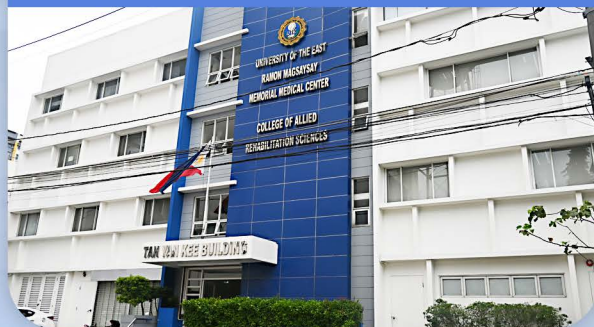
Exterior Wall Painting and Waterproofing of TYK December 15, 2024
