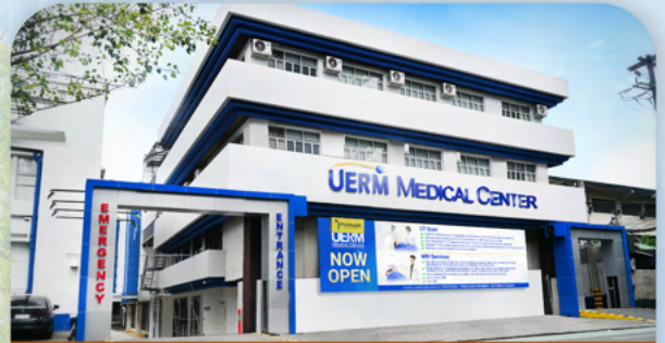
Renovation of Entrance & Exit Driveway with Complete Lighted Signages May 13, 2025
